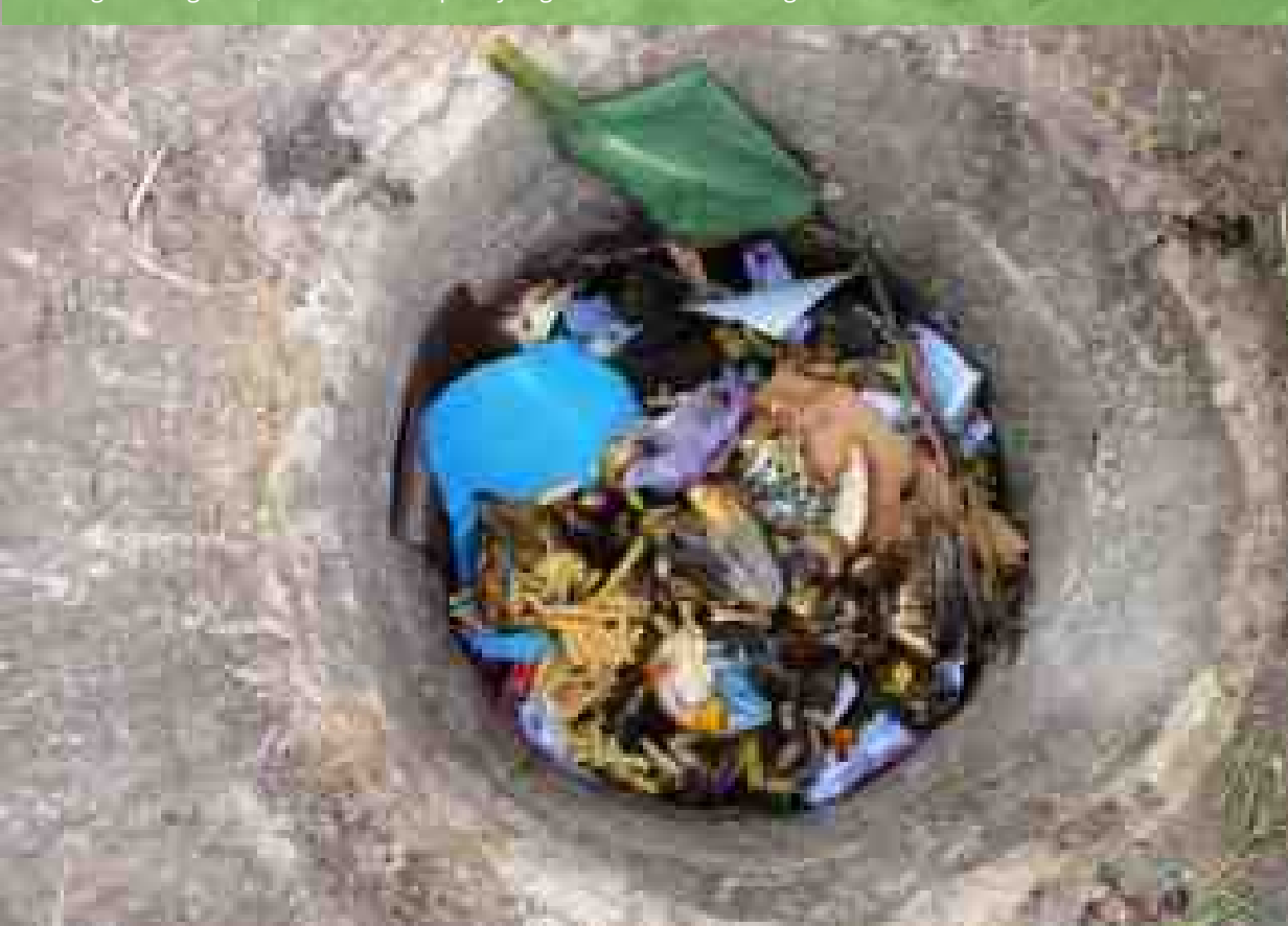
Feeding a biodigester, which can accept any organic material and degradable carbon. Susana Secretariat/Flickr
