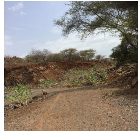
Livestock and people are impacted by open pits such as this one, which has been left by the extractive industry after taking materials for road construction. Edna Kaptoyo/GFC
