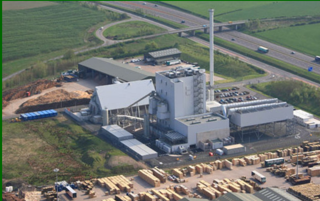
Photo: E.On's Steven's Croft biomass Power station in Scotland
