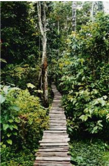
A suspended wooden road, constructed by the Uitoto indigenous community, Colombia. Photographer: Rodrigo Andrés Gamba Blanco
